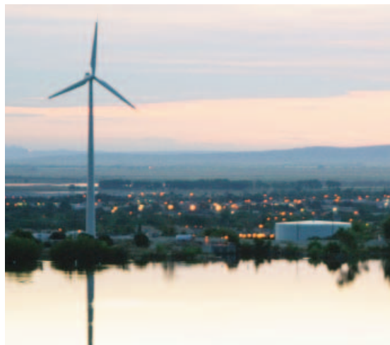
Palmdale Water District uses the power from this 950 kW turbine to provide electricity for the municipal water treatment plant 50 miles north of Los Angeles, California.
